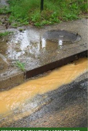
**SEDIMENT & POLLUTANT LADEN RUNOFF** FLOWS INTO STORM SEWER SYSTEMS.
