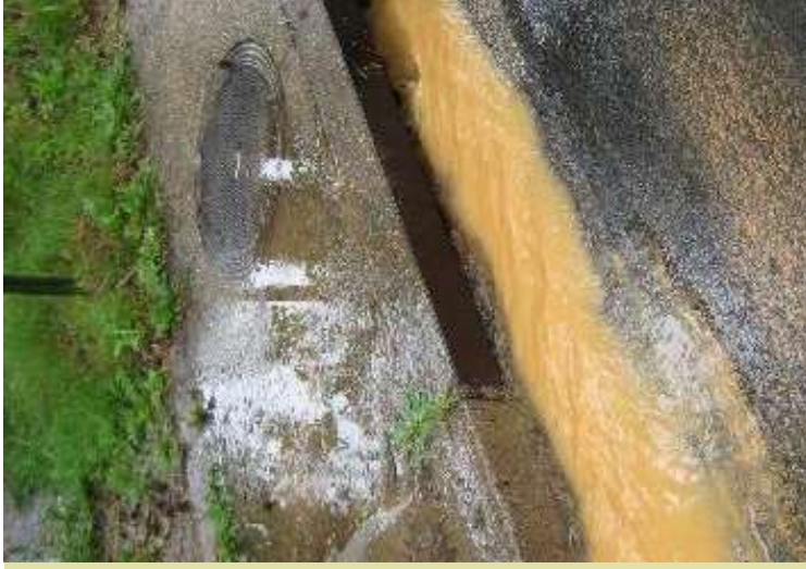
SEDIMENT & POLLUTANT LADEN RUNOFF FLOWS INTO STORM SEWER SYSTEMS.
